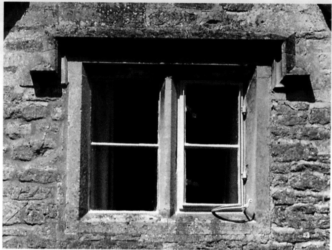
Fig. 6 Bibury (Glos.) A Cotswold two-light window with diamond- shaped mullion and drop-eared undercut hoodmould. 17th century. Photograph, author
